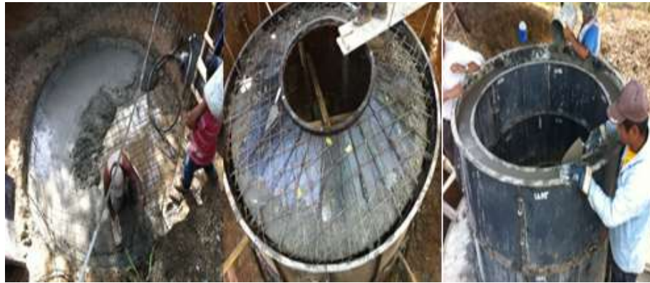
Figure 2. Construction phase. (1) Lenticular slab; (2) Stomach and shoulder; (3) Neck.
